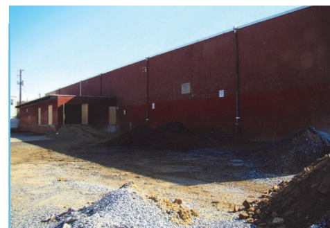
Construction has Begun
